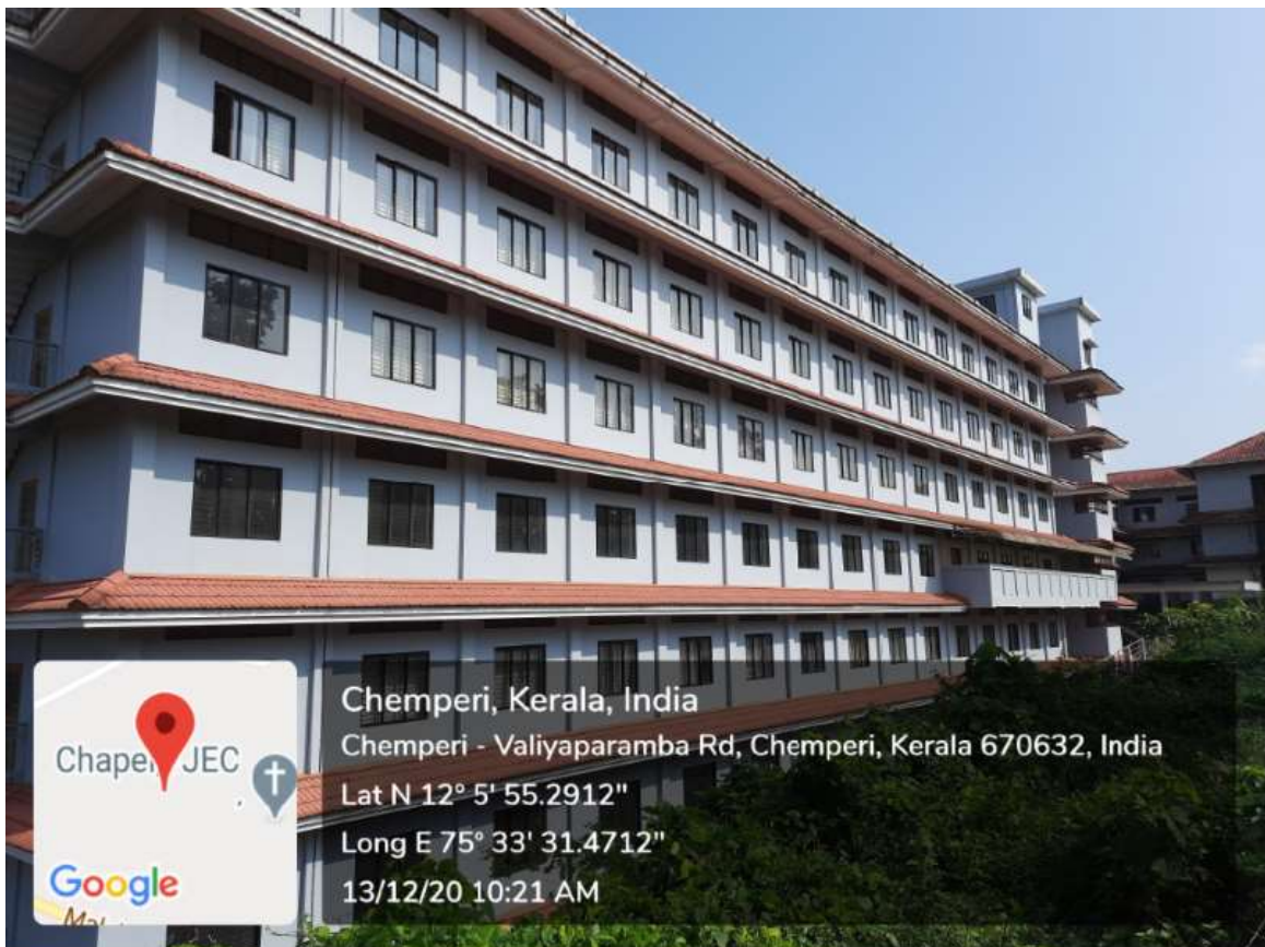
Figure: PG Hostel inside the campus- Side view: Top 4 floors are dedicated for PG Ladies with separate secure entrance.
